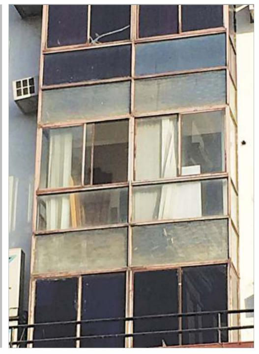
Normally at time of placing order for door & window, what is in your mind? In general practice we do emphasis more about the **COLOUR** not the grade of coatings. Using substandard powders and paints for exterior application will turn your window as above photographs.
